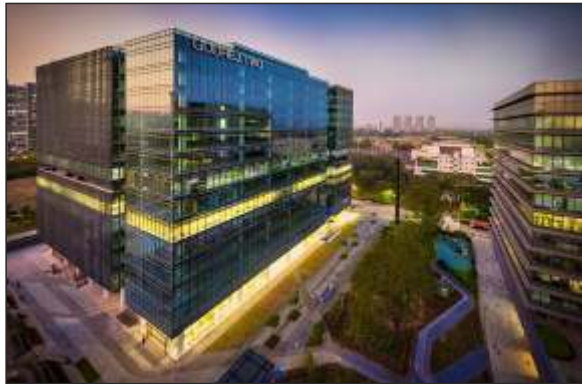
Godrej Two, Vikhroli 1.17 million sq.ft. Commercial Project with 50% equity stake
