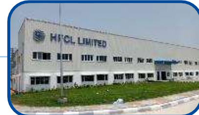
Optical Fiber Manufacturing Hyderabad, Telangana Capacity: Optical fiber - 6.4m fkm
