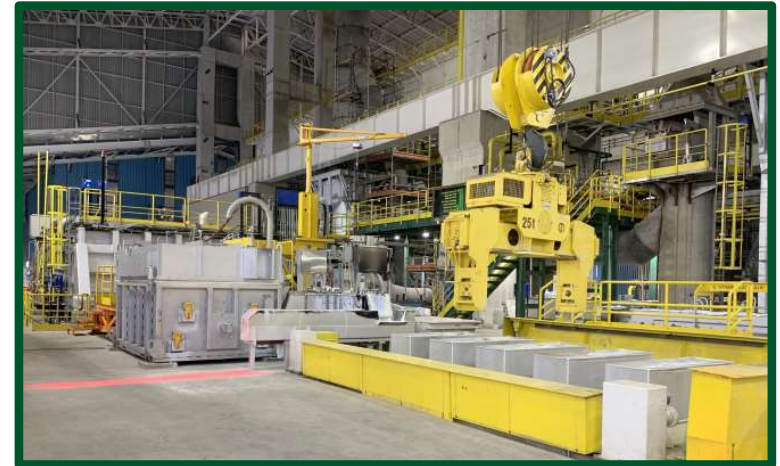
Casting pit in Pinda, Brazil
