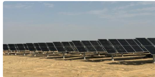
Modules installed at site
