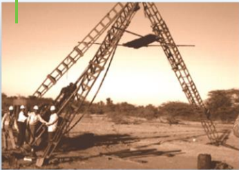
Conventional drill rig
