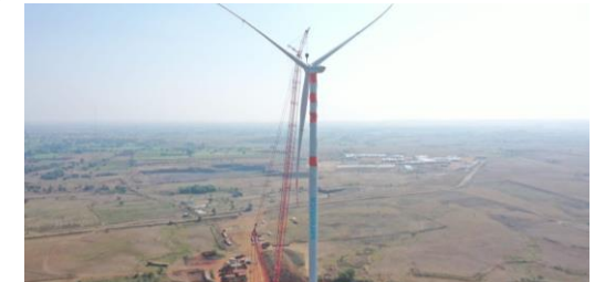
1st wind turbine installed
