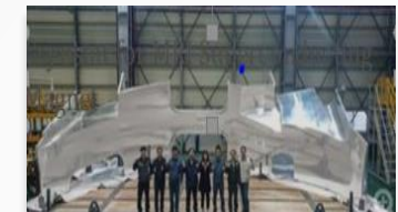
Thermal shield repair ITER Project
