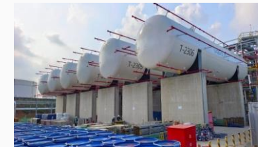
Hydrogen tank installation
