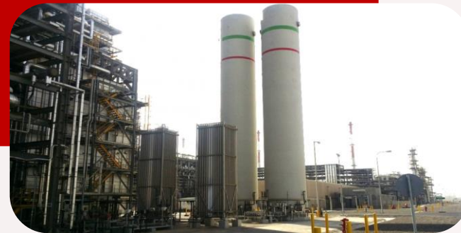
High Value order received for LIN Storage & Vaporiser system from Petrochemical industry for gulf country
