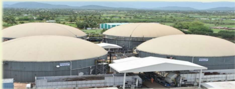
IndianOil's Biogas plant at Namakkal, Tamil Nadu
