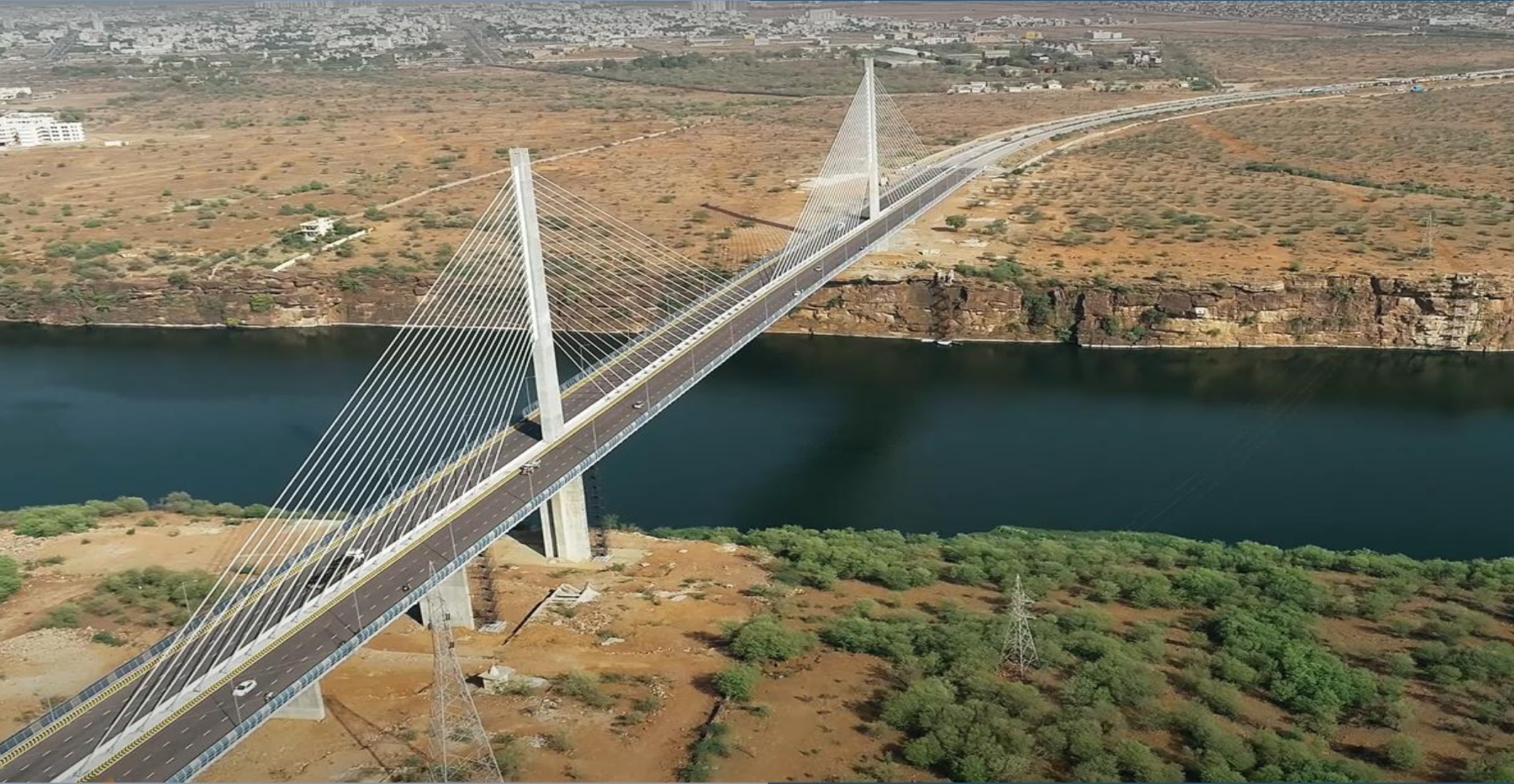
Cable Stayed Bridge on Chambal River near Kota
