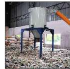
The ITC Limited facility for recycling MLP waste into plastic granules
