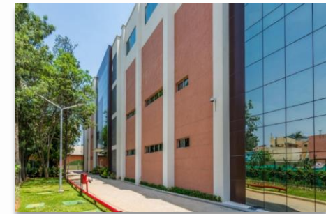
ITC Sankhya Data Centre, Bengaluru
