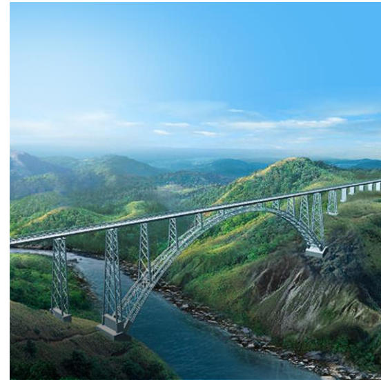
Chenab Bridge E410C high strength steel plates and HH 1080 rail
