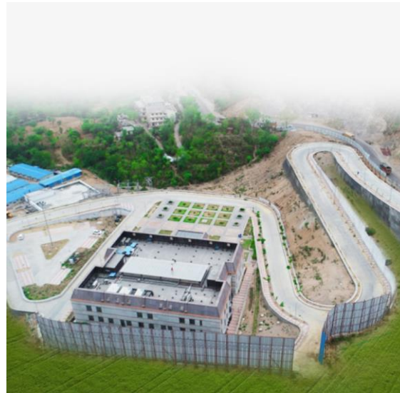
AIIMS Bilaspur, HP High strength fabricated structures
