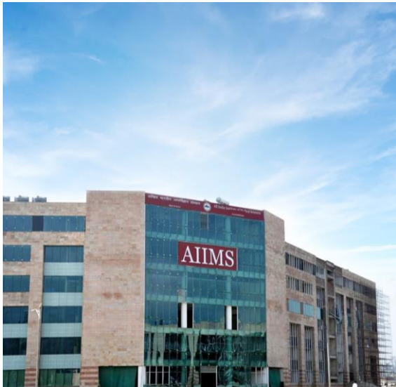
AIIMS Avantipura Pulwama, Kashmir High strength fabricated structures
