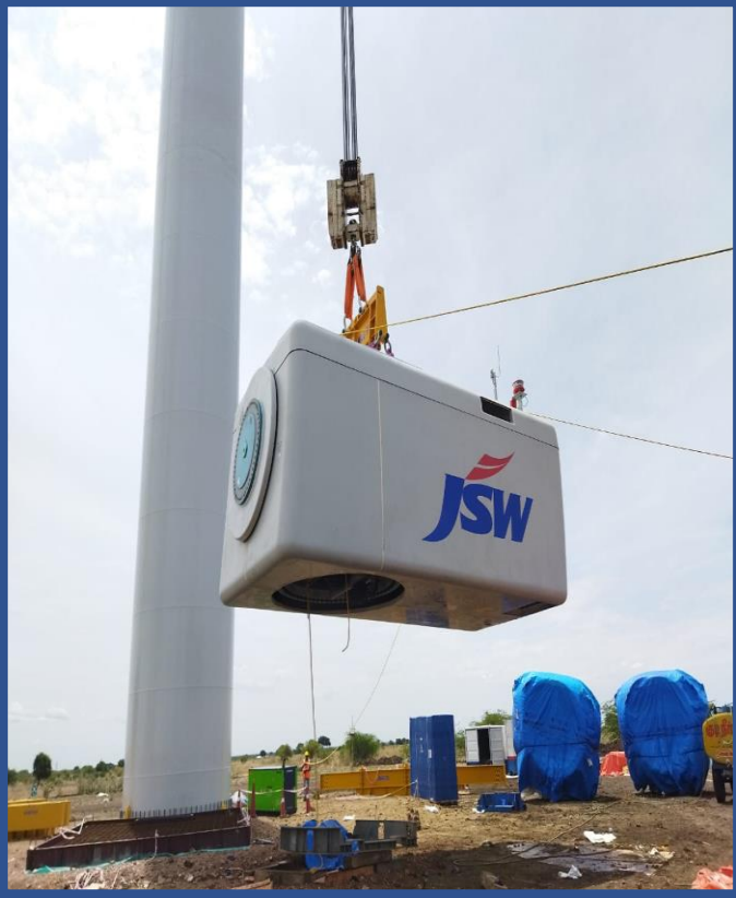
Nacelle Erection work in progress
