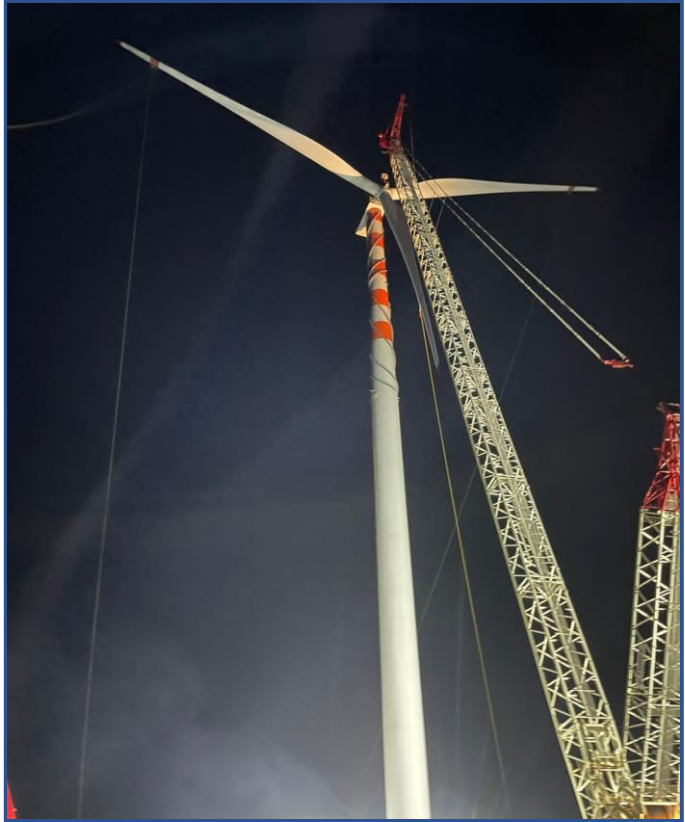
WTG Erection work in progress
