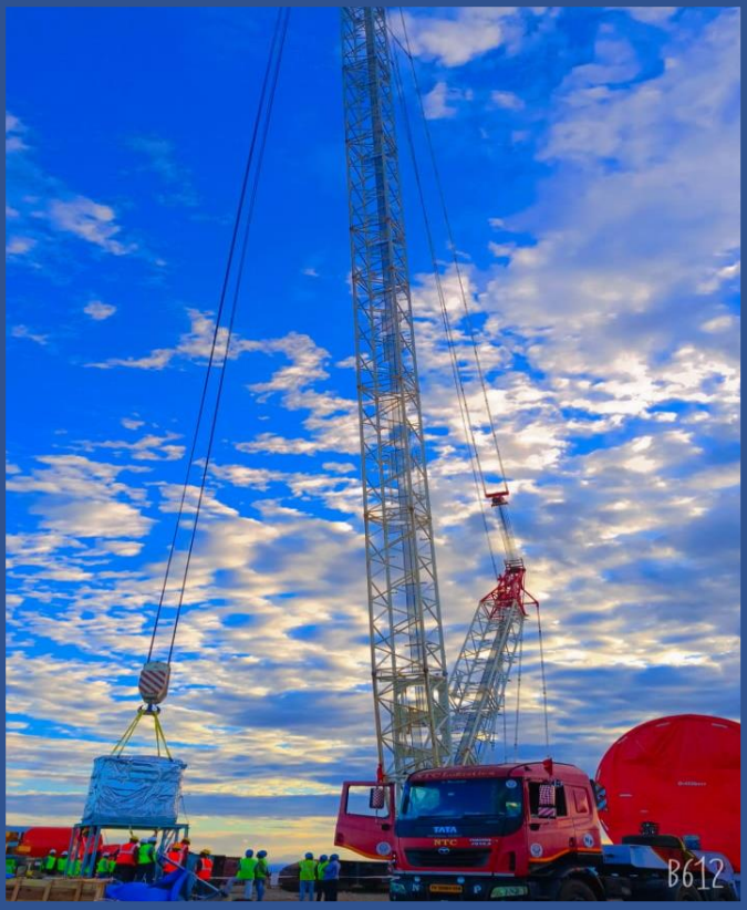
WTG Erection work in progress
