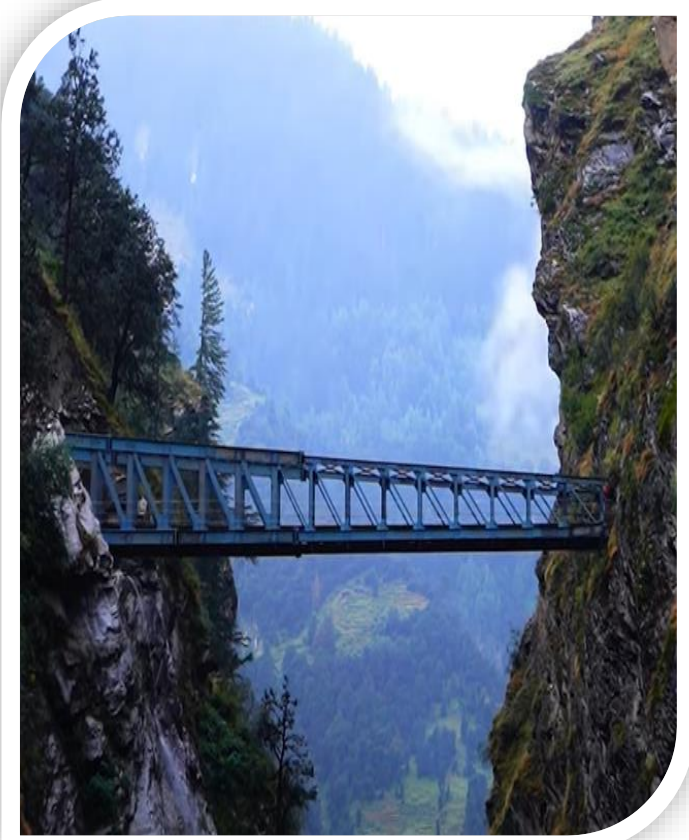
Steel Cantilever Bridge
