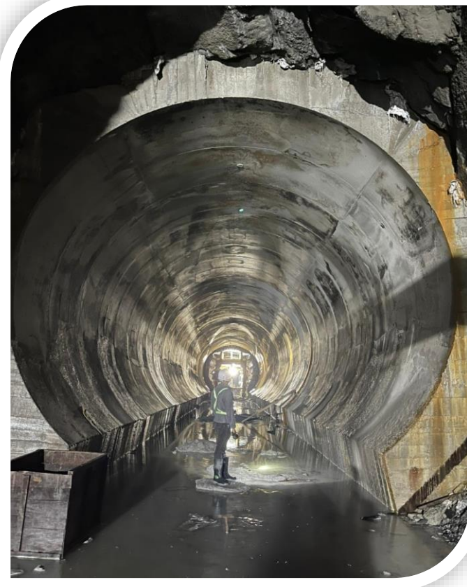
HRT Gantry Concrete Lining
