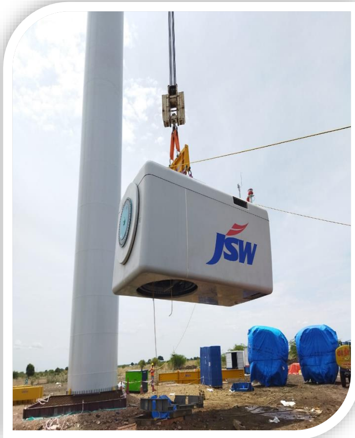
Nacelle and WTG erection
