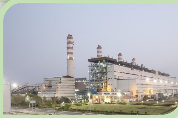
Green Belt & Plantation near Barmer Power Plant
