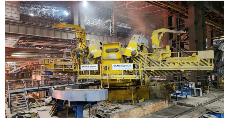
Ladle Turret at SMS-2 in BPSL
