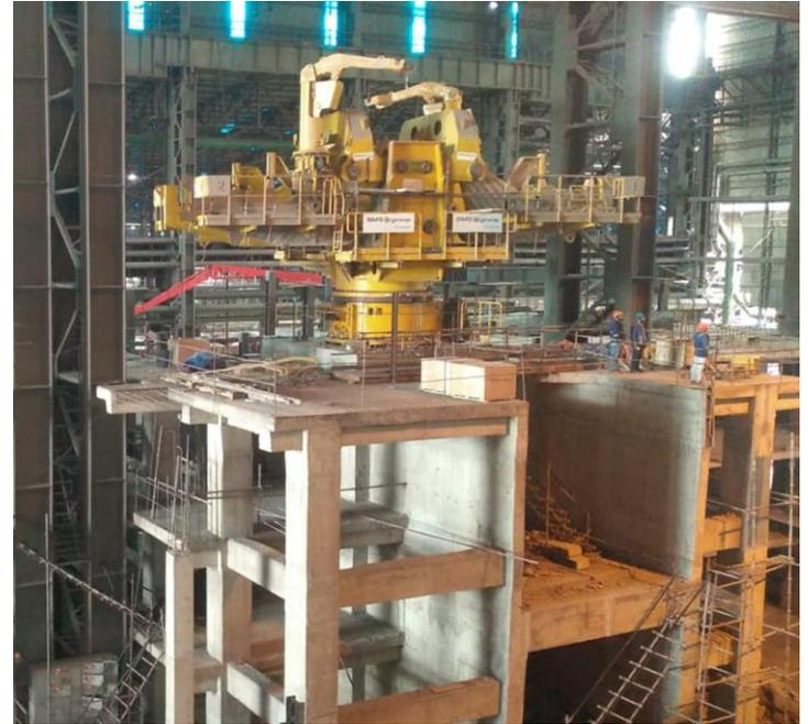
Ladle Turret & Casting Platform at SMS-2, BPSL Phase-II
