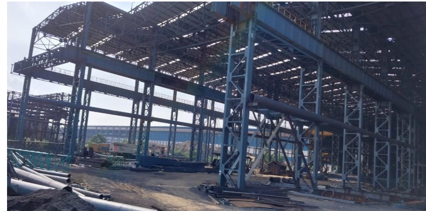
SMS-2 construction at BPSL
