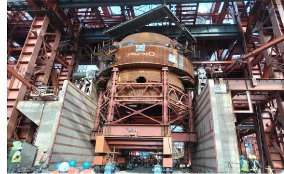
Converter vessel erected at SMS
