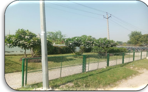
“Fencing and Maintenance work” was carried out at Garden near Goindwal Plant
