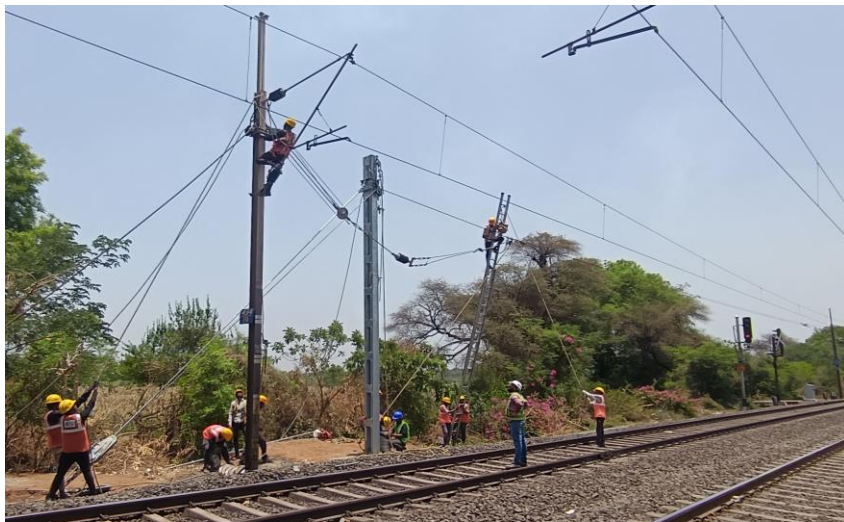
Speed upgradation project, Vadodara-Godhra (Part of Bombay Delhi section)
