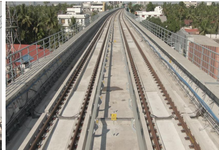
Ballastless track works, Kochi Metro
