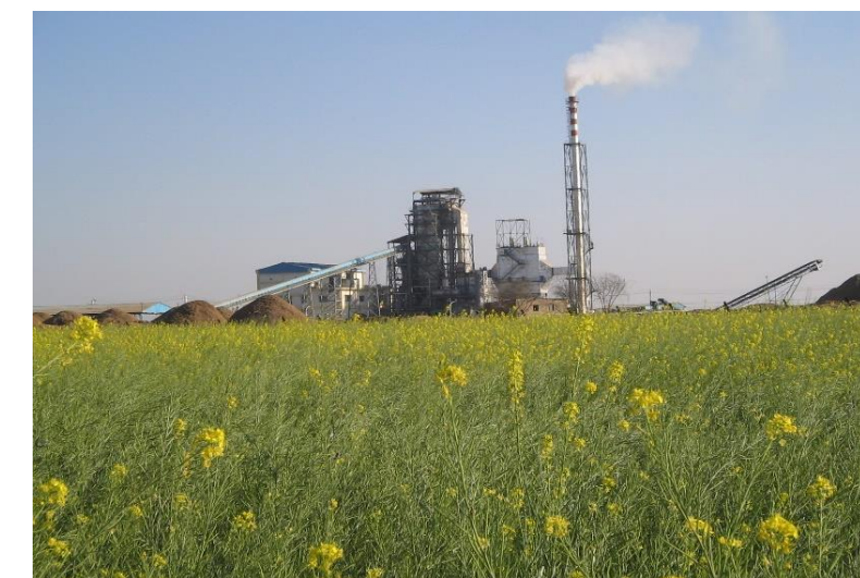
Uniara Power Plant, Rajasthan (India)
