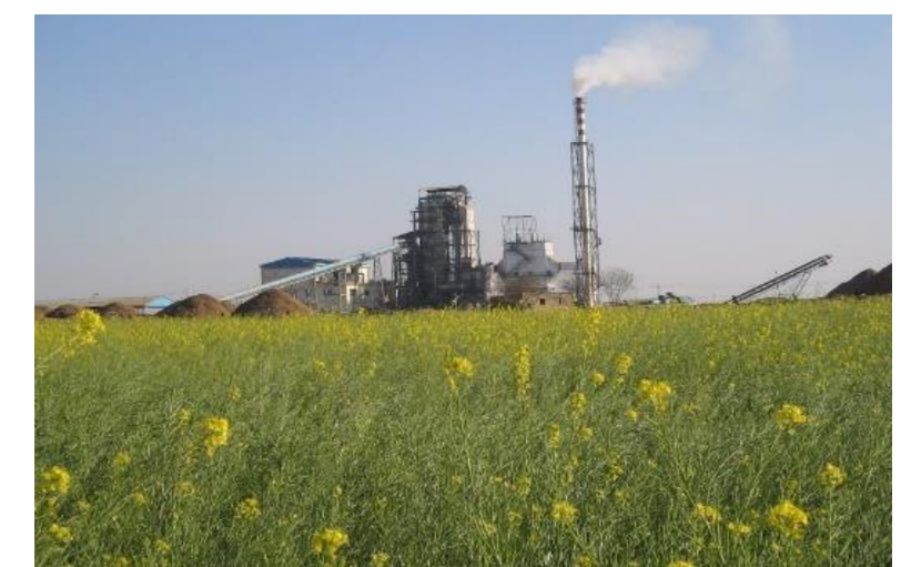
Uniara Power Plant, Rajasthan (India)
