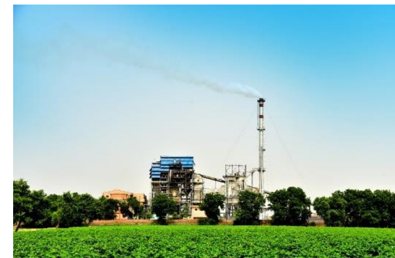
Padampur Power Plant, Rajasthan (India)
