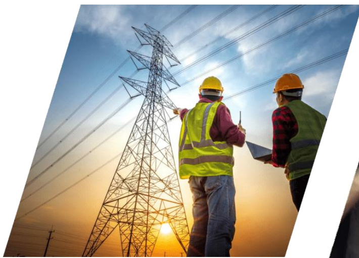
Power Transmission & Distribution
