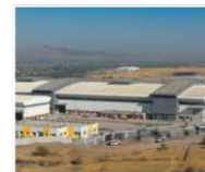
Energy Pumps Division, Shirwal
