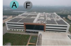
Unit-2, Atchutapuram 10Bn units, 161 KL
