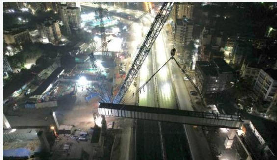
Elevated Corridor work in full-swing
