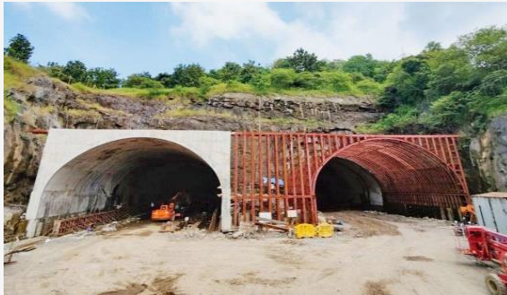
Tunnel entry and exit points near completion
