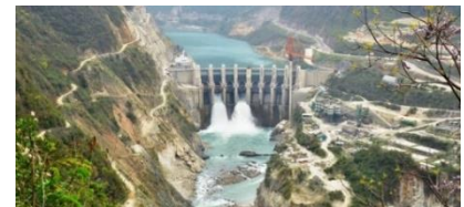
Srinagar Hydro Electric Plant
