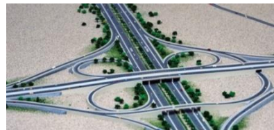
Sheikh Khalifa Interchange, UAE
