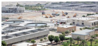
Water Treatment Plant, Doha
