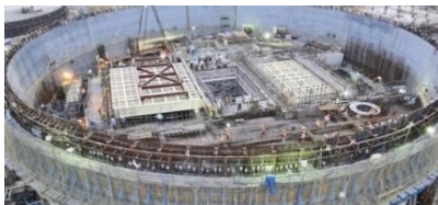
Kakrapar Nuclear Power Plant, Guj
