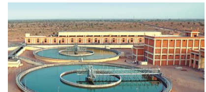
Water Treatment Plant, Barmer
