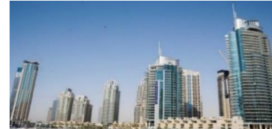
Twin Towers, Dubai Marina
