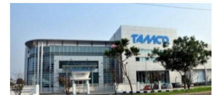
MV Switchgear Factory, Malaysia
