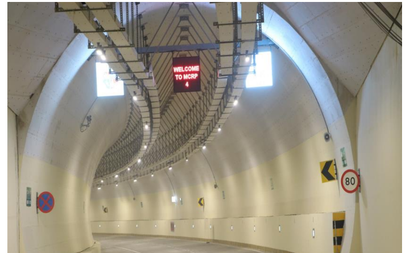
Mumbai Coastal Road Project
