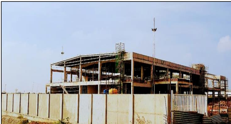
Nissei facility under construction at Origins Chennai
