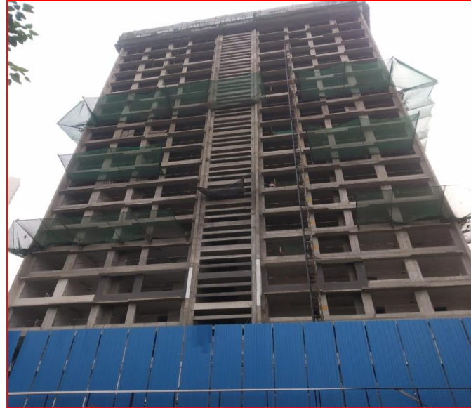
Roots: Site under construction
