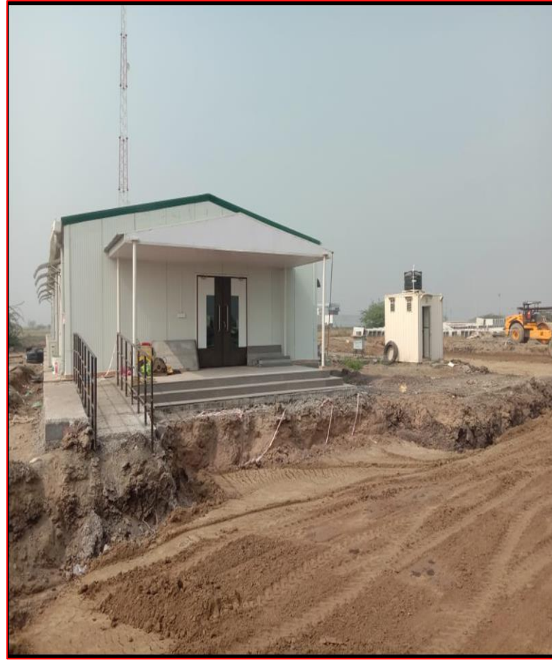
Site Under construction, Ahmedabad
