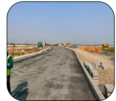
Under Construction Site
