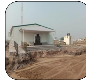
Under Construction Site
