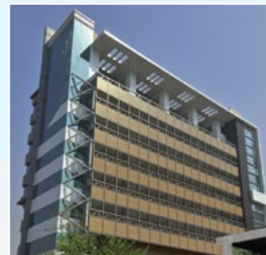
Airtel Switching & Data Centre - Navi Mumbai
