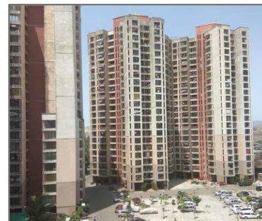
Rehab Buildings – Tata Housing
