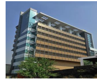
Airtel Mobile Switching & Data Centre
