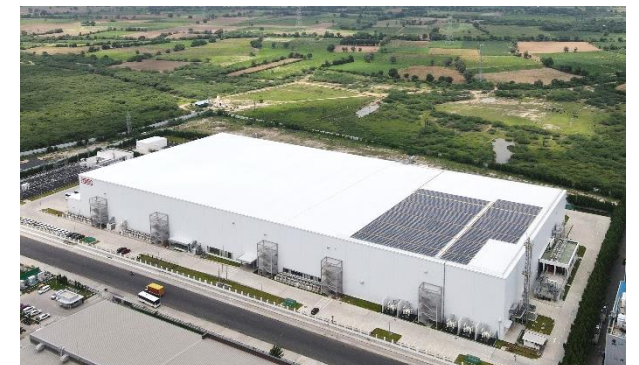
TDS Lithium-Ion Battery Gujarat Pvt. Ltd.
