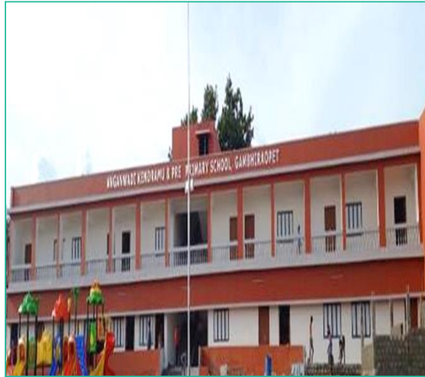
Establishing a school with a capacity of 400 students in Gambhiraopet, Telangana
