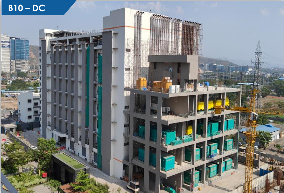
Completed and Handed over block to the client
