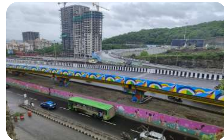
Chandni Chowk Flyover, Pune
