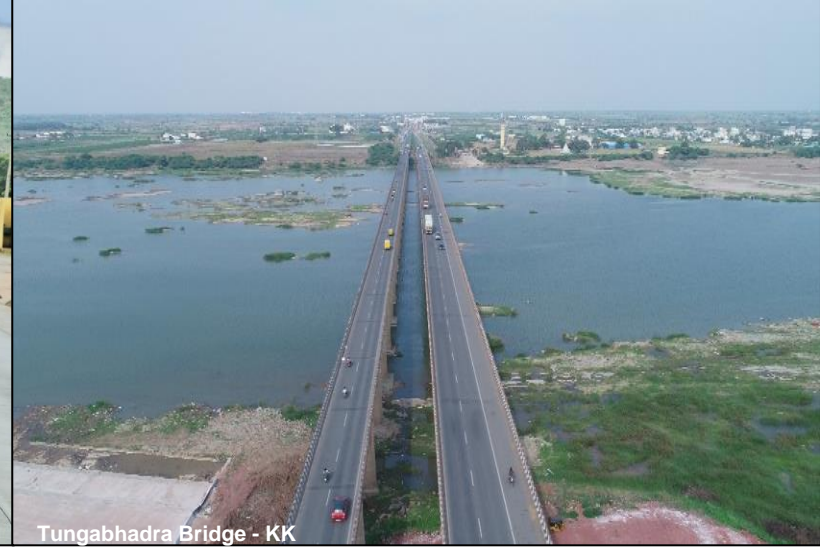
Tungabhadra Bridge - KK
