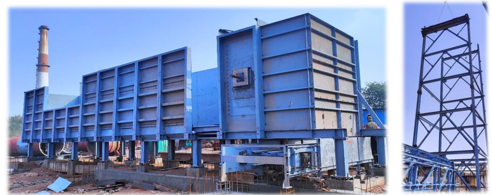
Erection of Alternative Fuel Feeder and Transfer Tower at Nimbol
