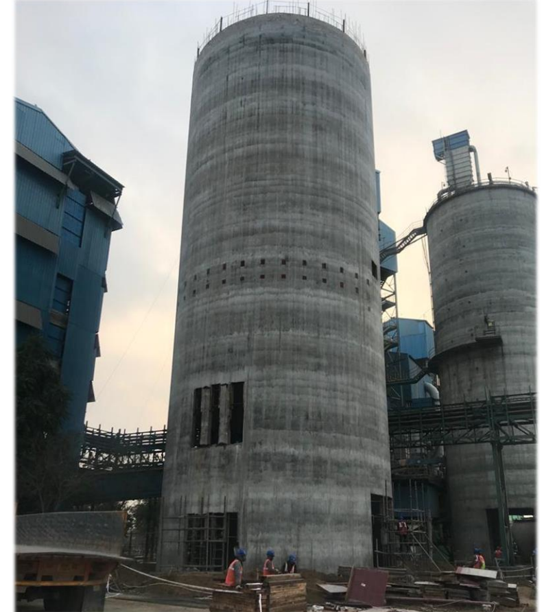
Cement Silo, Bhiwani Cement Plant
