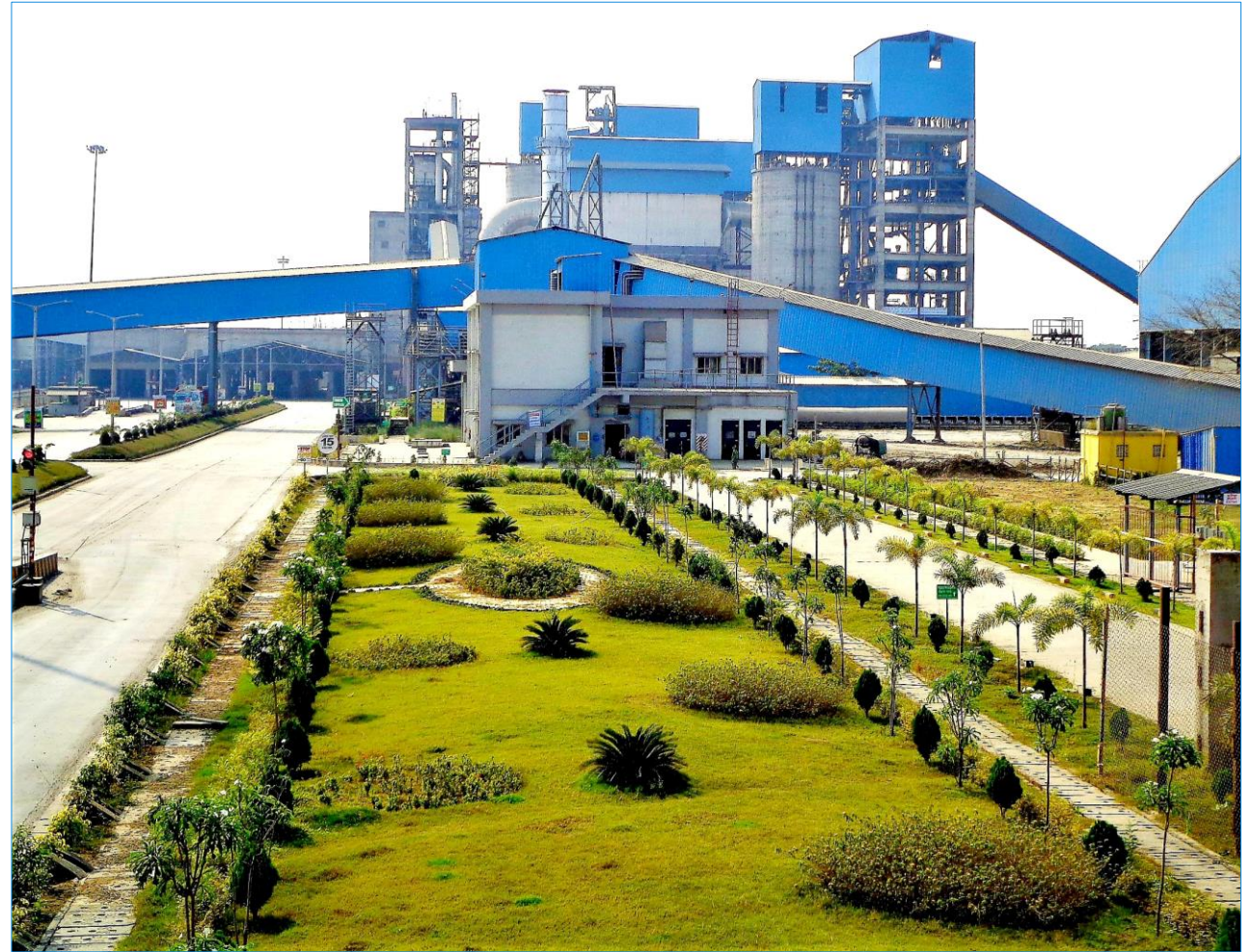
Panagarh Cement Plant
