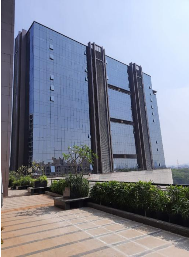
Tower 2 – Construction Completed, OC Received
