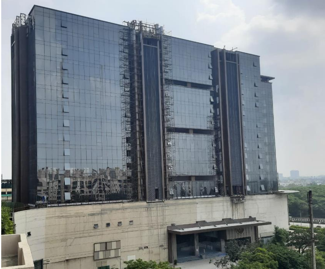
Tower 2 – Construction Completed, OC Received
