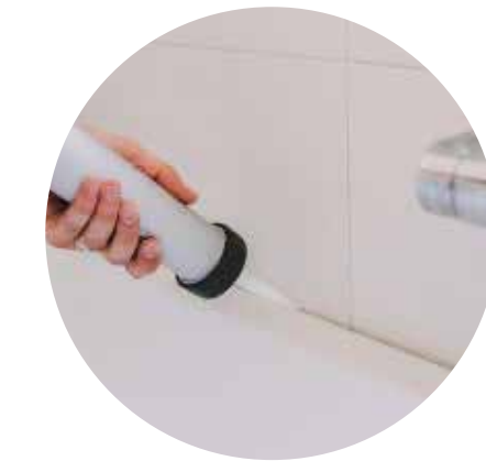
Sanitary gap filling
