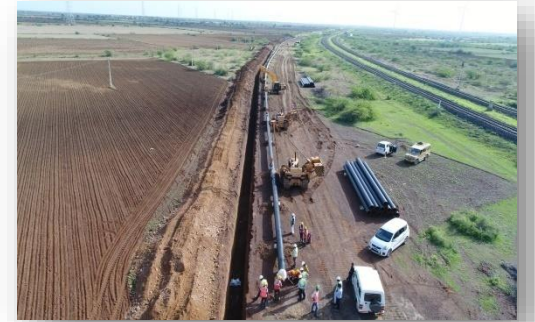
Lowering of pipe at Mundra to Kandla pipeline project-90 KM, Adani
