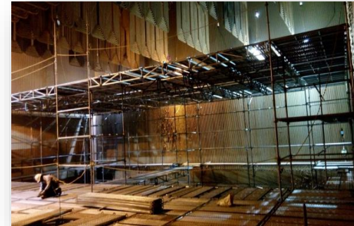
Cuplock Scaffolding Erection 800 MW, Mundra
