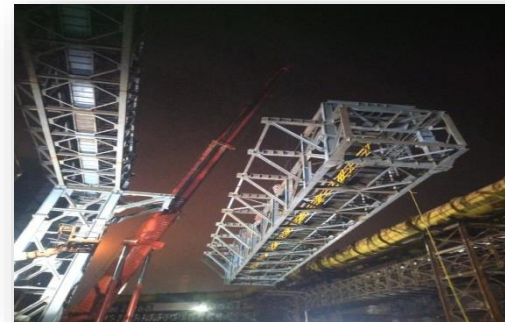
Utility Corridor, Gallery Erection, Dolvi, JSW
