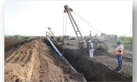
Lowering of Pipe Section, Mundra, Adani
