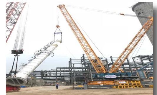
Urea Reactor Tank Installation At Ramagaundam, Telangana
