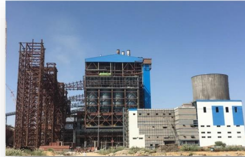
2x660 MW Suratgarh STPP, RRVUNL
