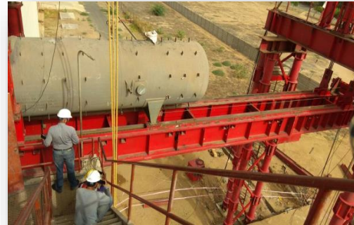
HP Heater Replacement 800 MW, CGPL Mundra 2
