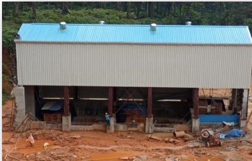
Implementation of Hydro Electric Project (2MW/5.14 Mu)-KSEB
