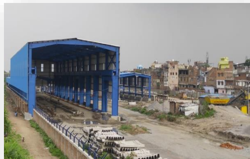
MEMU Shed at Kanpur-RVNL
