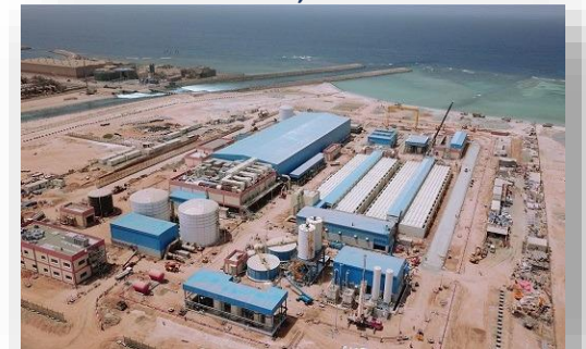
Second Water Expansion Seawater Desalination Plant, Shuaibah-3, FISIA ABEIMA, KSA
