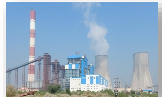
2x660 Mw STPS, Suratgrah - RRVUNL
