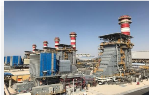
1,519 MW Fadhili CHPP, Doosan, KSA
