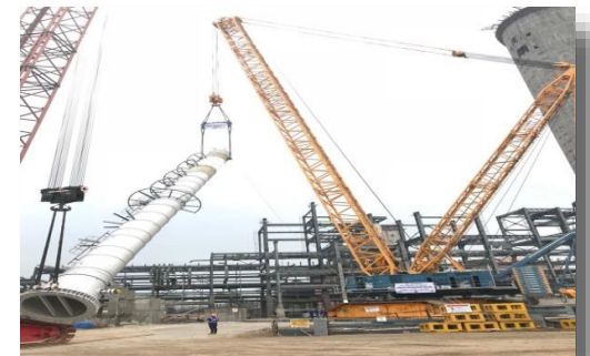
Urea Reactor Tank Installation At Ramagaundam, Telangana
