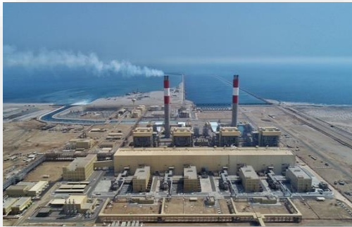
4X660 MW Shuqiaq SSPP, KSA (Completed Project)
