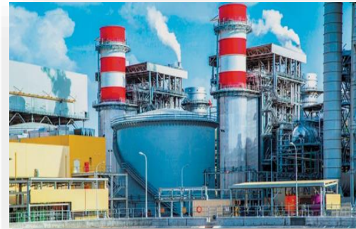
1,516 MW IBRI IPP, SEPCO – 3, Oman (Completed Project)
