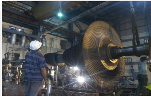
Capital Overhauling of Turbine 63 MW, SV Power, Korba Rotor Lifting-3
