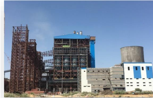
2x660 MW Suratgarh STPP, RRVUNL
