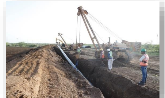
Lowering of Pipe Section, Mundra, Adani
