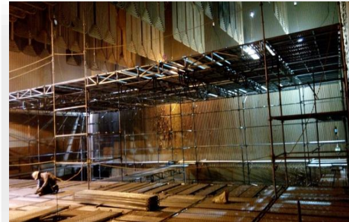
Cuplock Scaffolding Erection 800 MW, Mundra
