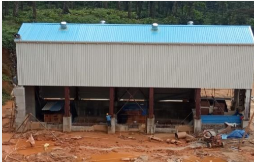
Implementation of Hydro Electric Project (2MW/5.14 Mu)-KSEB
