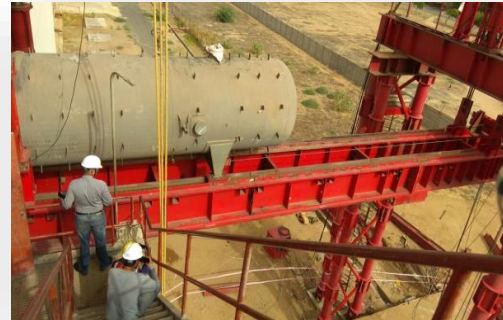
HP Heater Replacement 800 MW, CGPL Mundra 2
