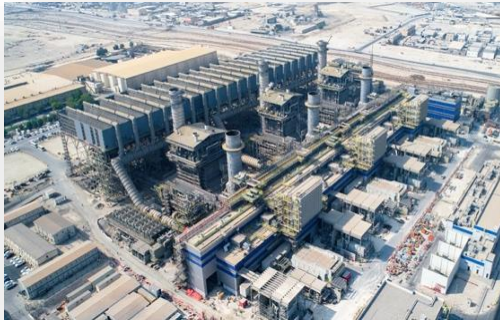
1,800 MW Alba PS5 CCPP, Bahrain (Completed Project)
