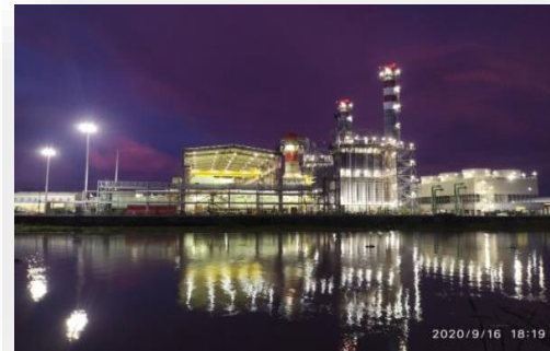
220 MW (GAS) / 212 MW, (HSD) CCPP, Bisho Infra, Bangladesh
