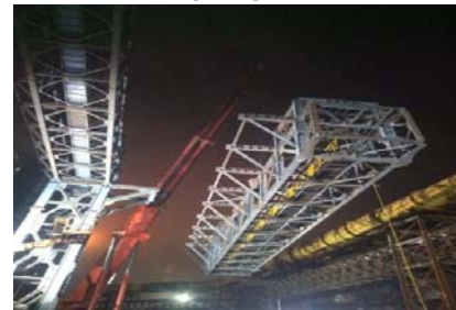
Utility Corridor, Gallery Erection, Dolvi, JSW
