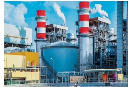
1,516 MW IBRI IPP, SEPCO – 3, Oman (Completed Project)
