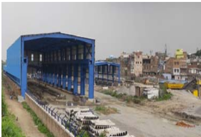
MEMU Shed at Kanpur-RVNL
