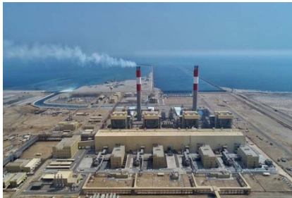
4X660 MW Shuqiaq SSPP, KSA (Completed Project)
