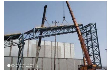
Erection of P&N Gallery at Bellary, JSW
