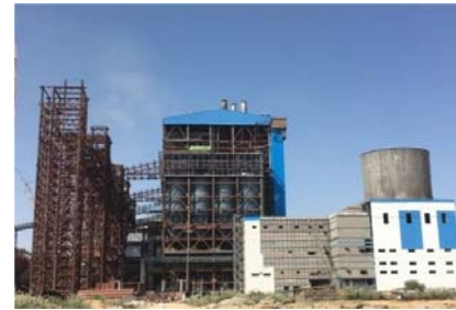
2x660 MW Suratgarh STPP, RRVUNL
