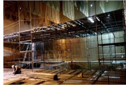
Cuplock Scaffolding Erection 800 MW, Mundra
