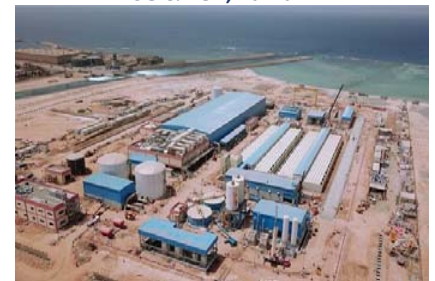
Second Water Expansion Seawater Desalination Plant, Shuaibah-3, FISIA ABEIMA, KSA
