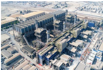
1,800 MW Alba PS5 CCPP, Bahrain (Completed Project)
