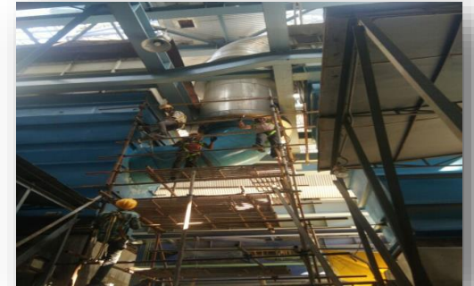
MSH Line Modification, 600 MW Singareni
