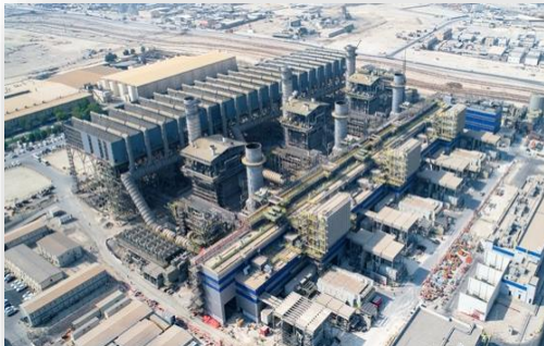
1,800 MW Alba PS5 CCPP, Bahrain (Completed Project)
