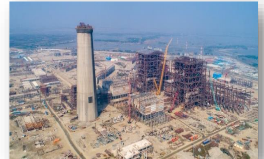
2X660 MW at Rampal, Maitree, Bangladesh-BIFPCL
