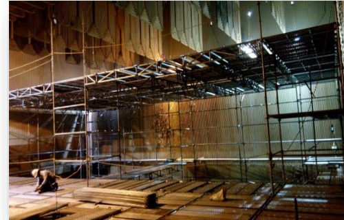
Cuplock Scaffolding Erection 800 MW, Mundra
