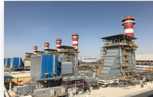
1,519 MW Fadhili CHPP, Doosan, KSA
