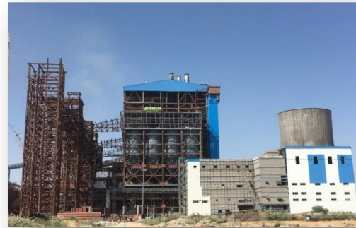
2x660 MW Suratgarh STPP, RRVUNL
