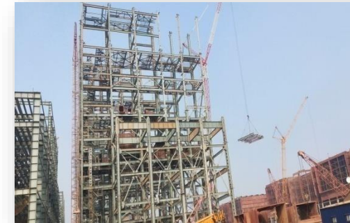
5x800 MW Yadadri TPP, TSGENCO
