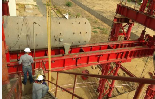
HP Heater Replacement 800 MW, CGPL Mundra 2
