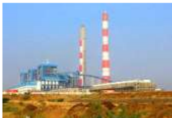
3X800 MW, BOILER, ESP, PIPING, STG KUDGI, DOOSAN, L&T & TOSHIBA
