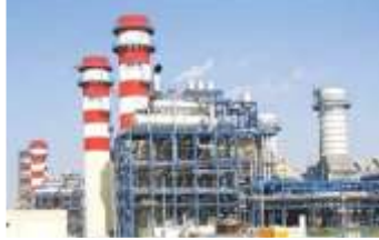
2X157 MW GT POWER PLANT, LIBYA (COMPLETED)
