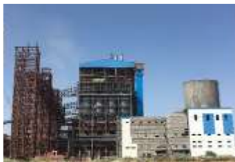
2X660 MW STPP, BOILER , ESP, STRUCTURE & STG U#7&8, SURATGARH, BHEL
