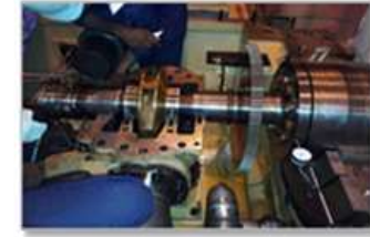
228MW, STEAMTURBINE,SABIYA, KUWAIT, MAIN OIL PUMP OVERHAULING
