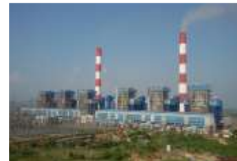
BOILER, ESP, STRUCTURE, TG AUXILIARIES,UMPP 6X660MW, SASAN, R INFRA (COMPLETED)
