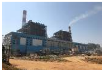
2X660 MW IBTPS, STRUCTURE & STG, BANHARPALLI, BHEL
