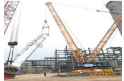
UREA REACTOR TANK INSTALLATION AT RAMAGAUNDAM, TELANGANA
