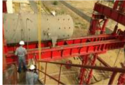
HP HEATER REPLACEMENT 800MW ,CGPL MUNDRA2
