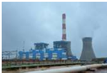
2X600MW TPP, BOILER & STG, MANGALORE, LANCO (COMPLETED)
