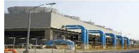
Infrastructure Construction (Civil)
