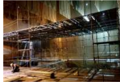
CUPLOCK SCAFFOLDING ERECTION 800MW,MUNDRA
