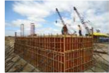
1X110 MW, CIVIL AND STRUCTURAL WORKS ,R&M OF MAIN PLANT, BATHINDA, BHEL (COMPLETED)
