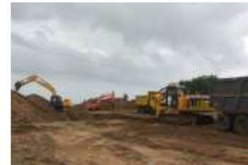
KALWESHWARAM CANAL PROJECT, 54 KM RAMAYAMPET
