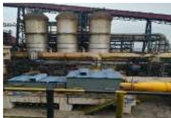
BLAST FURNACE, STEEL PLANT WORK, JSPL, ANGUL
