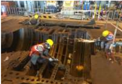
MAIN TURBINE OVERHAULING ,660 MW KAWAI
