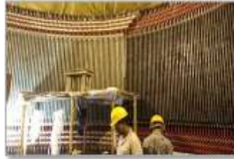
6X200 MW HEP, BHUTAN INSTALLATION OF HYDRO TURBINE & GENERATOR
