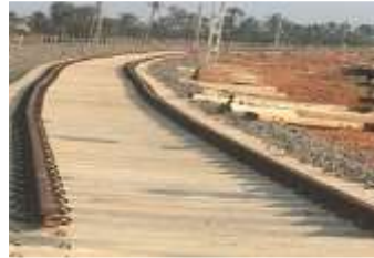
GDV-MTM 37 ,DOUBLING & ELECTRIFICATION WORKS , RVNL
