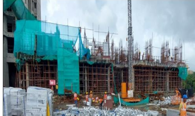
TOWER - 5 : 2nd slab WIP
