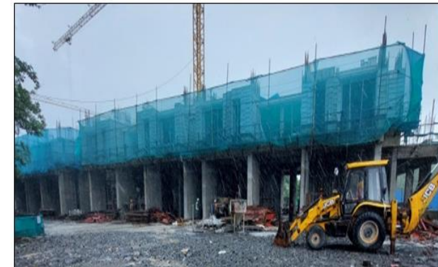
TOWER - 6 : 2nd slab WIP
