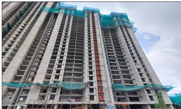
TOWER - 4 : 30th slab WIP
