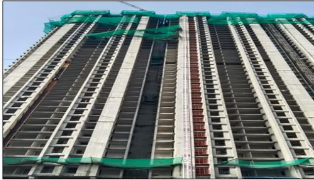
TOWER - 1 : 42nd slab ready to cast
