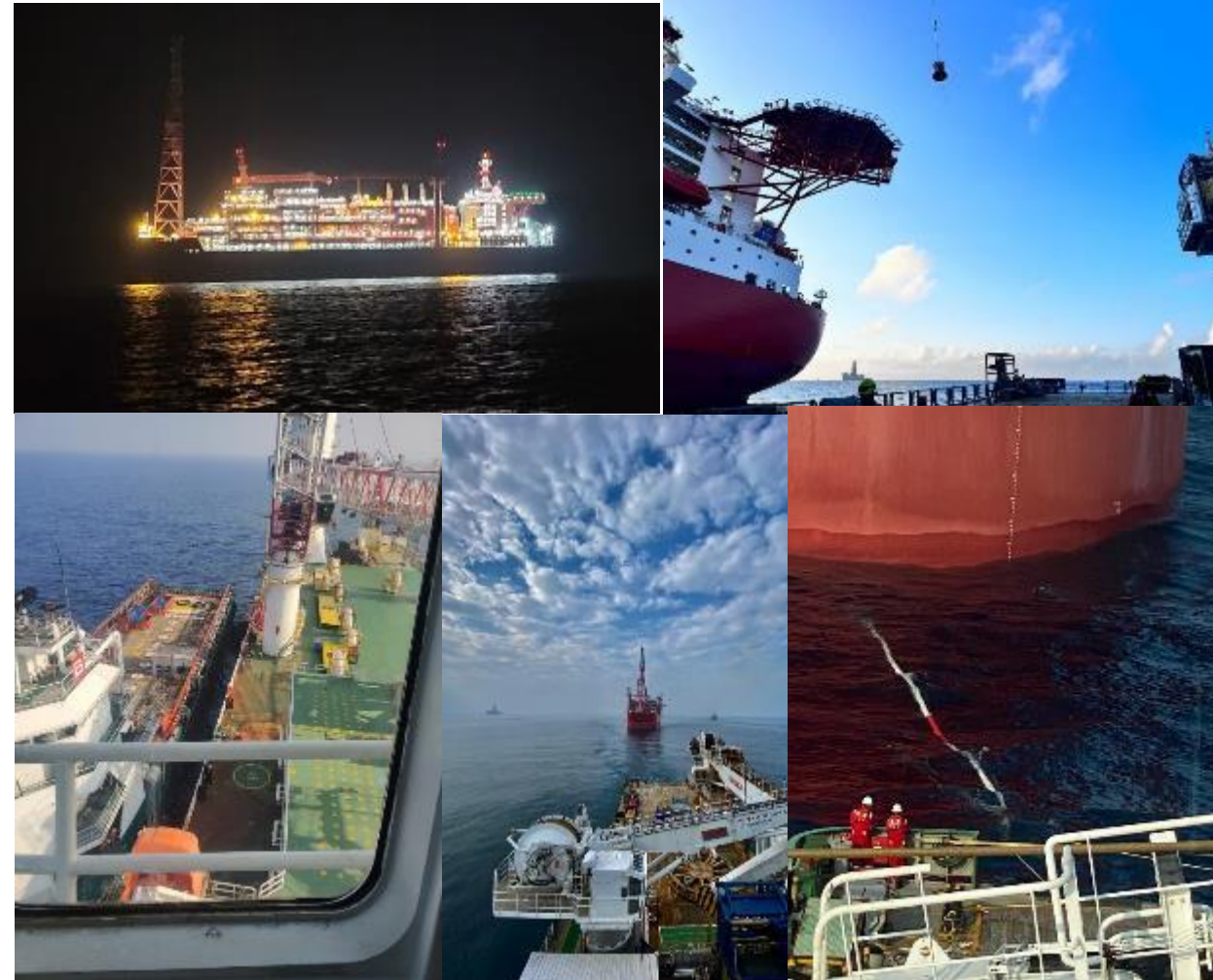
MJ FPSO Hookup & Field Installation Pictures
