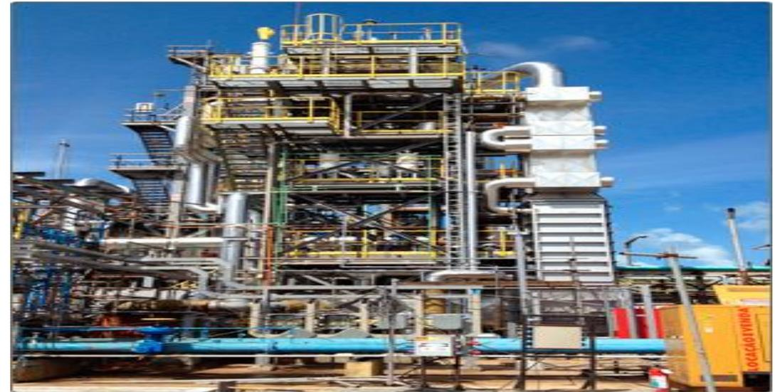
Power generated by using flu gases and capturing of heat through waste heat recovery boilers
