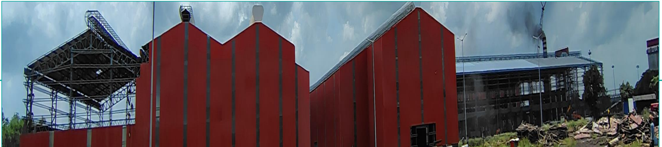
Cold and Hot trial runs have begun
