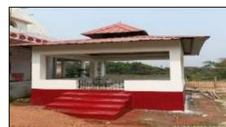
PUBLIC UTILITY AREA CONSTRUCTION
