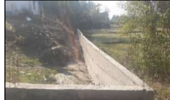
BOUNDARY WALL CONSTRUCTION
