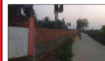
CONSTRUCTION OF WALL
