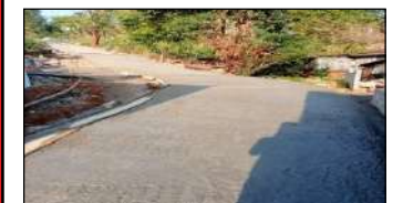
CONSTRUCTION OF RCC ROAD
