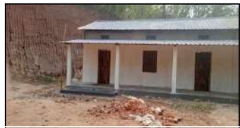
SCHOOL BUILDING RENOVATION
