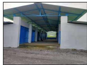
CONSTRUCTION OF LOCAL MARKET
