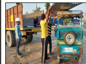
CGI SHEET DISTRIBUTION AFTER MASSIVE STORM
