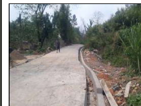
CONSTRUCTION OF ROAD
