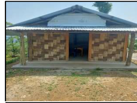
NEW SCHOOL SHED CONSTRUCTED
